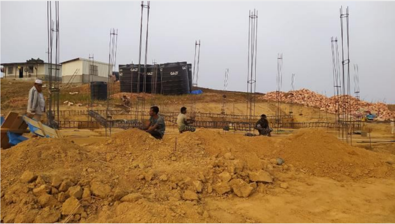
Rod binding work for grade beam at guest on 21-01-21
