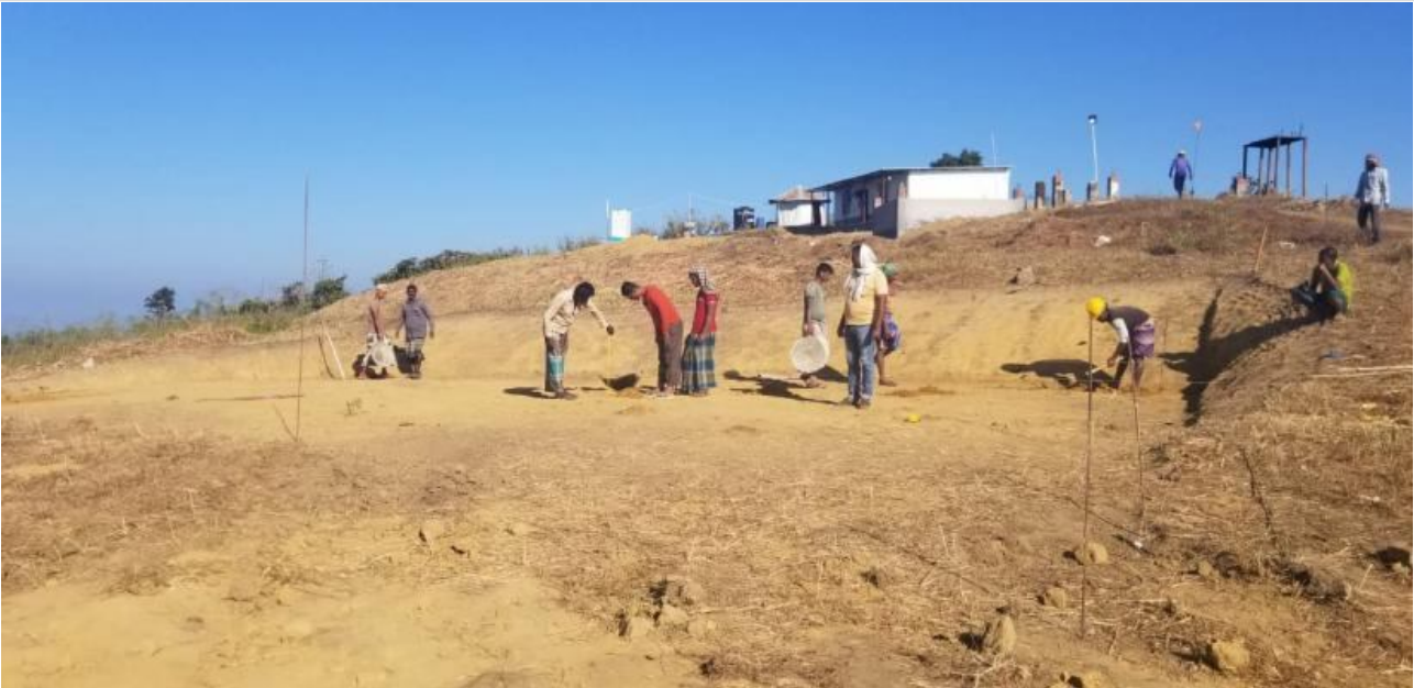
Guest House-Preparation for Layout on 07-01-21
