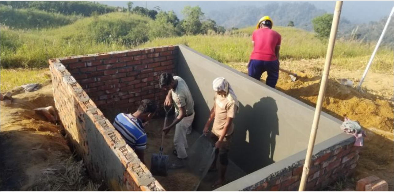
Plaster work for labour Shed on 12-01-21
