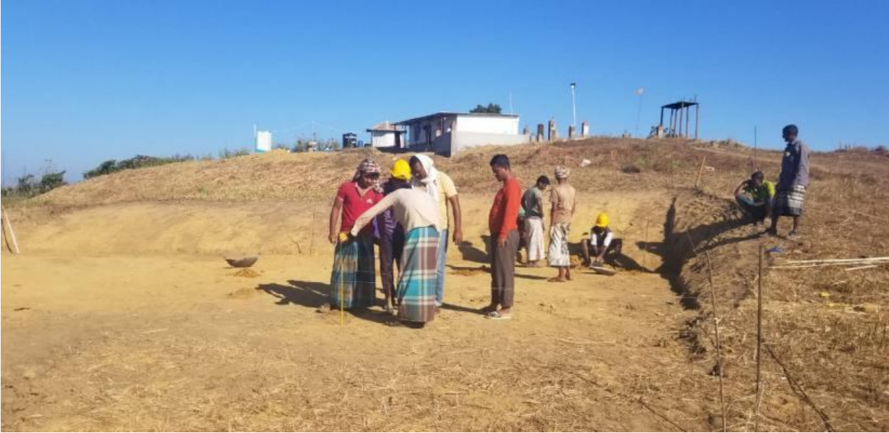
Guest House-Preparation for Layout on 05-01-21
