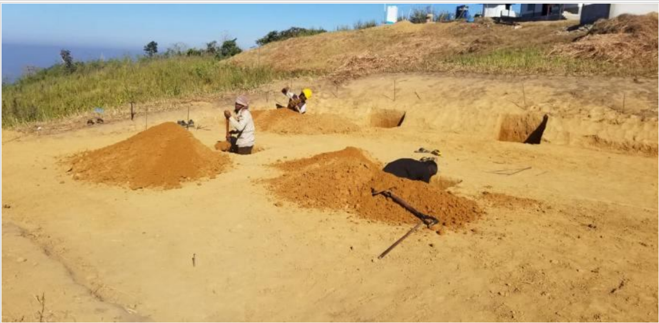
Guest House-Excavation on 09-01-21
