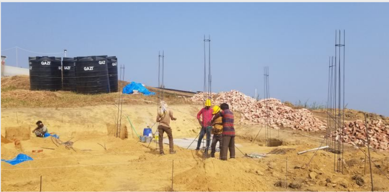
Column standing work on going at G.House on 14-01-21
