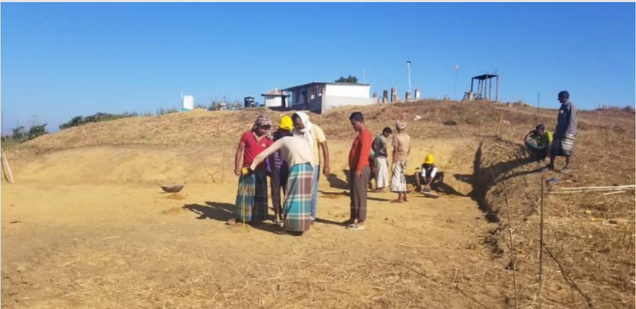
Guest House-Preparation for Layout on 06-01-21
