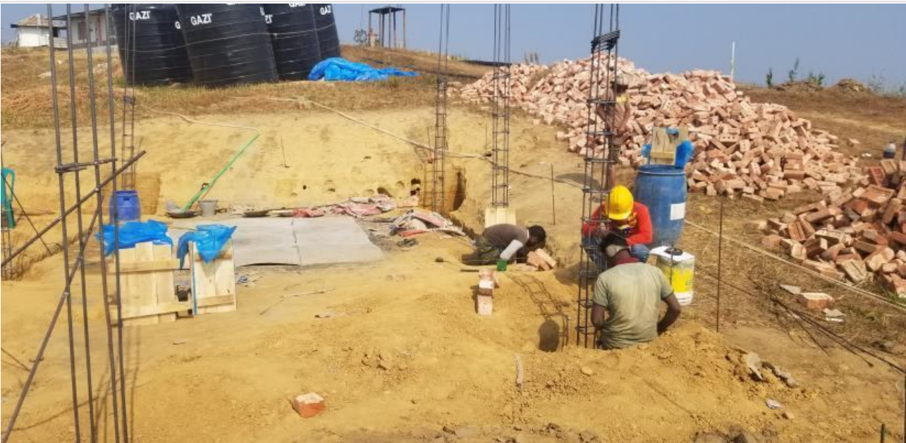
Shuttering fitting work for short column on 16-01-21
