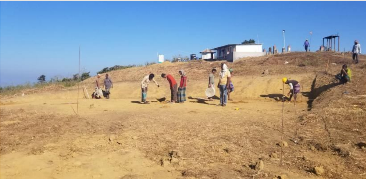
Guest House-Preparation for Layout on 05-01-21
