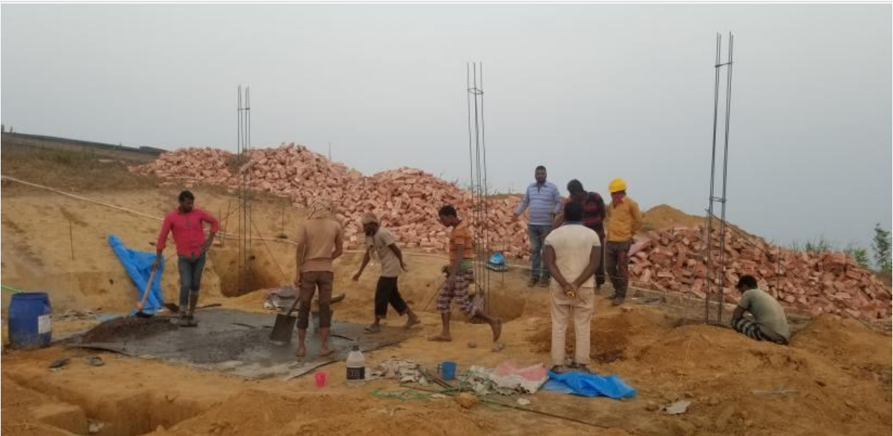
Footing & column casting work on going on 13-01-21
