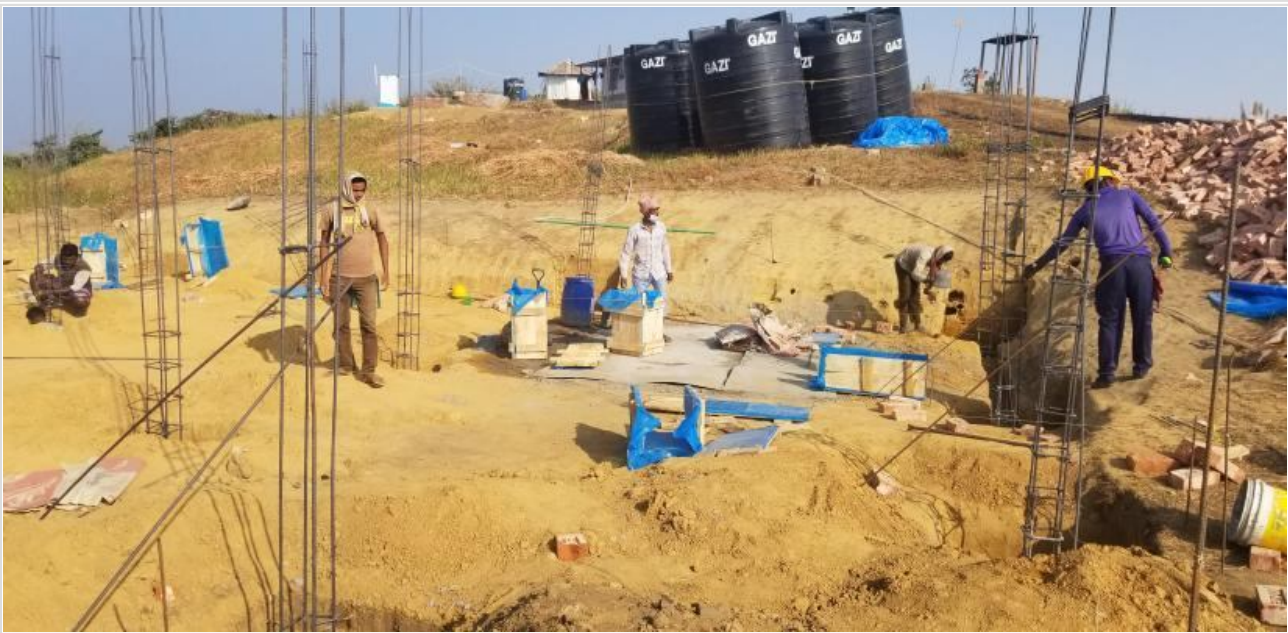
Shuttering fitting work for short column on 17-01-21
