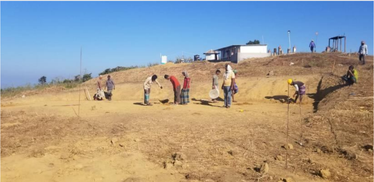
Guest House-Preparation for Layout on 06-01-21
