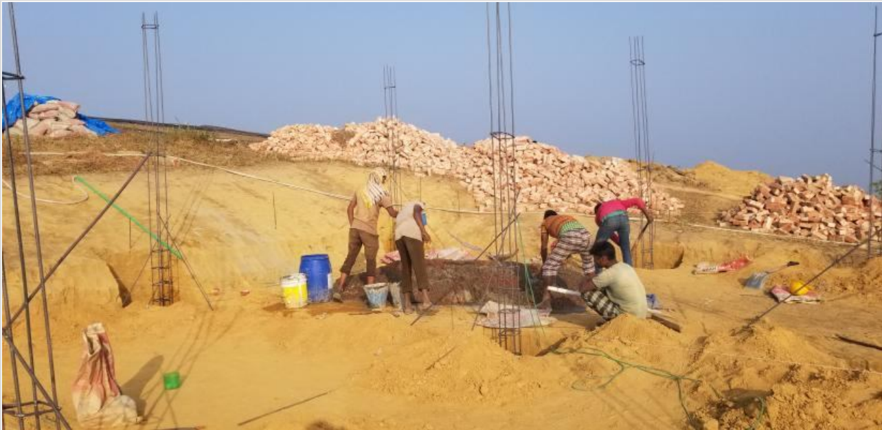
Footing & column casting work on going a on 14-01-21
