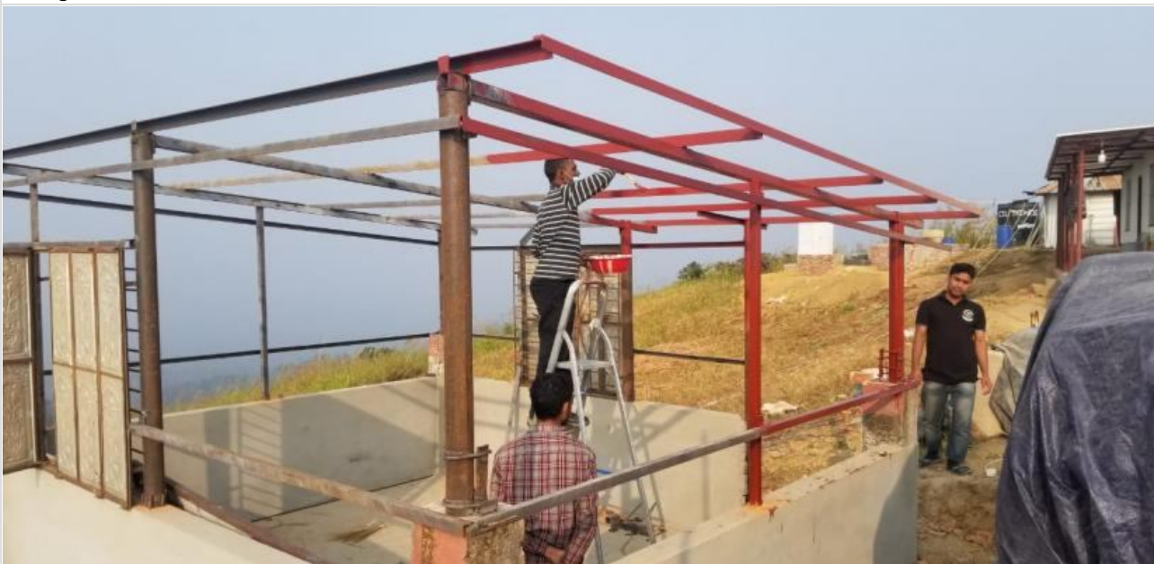
Mechanics Shed Frame Work on 20-01-21
