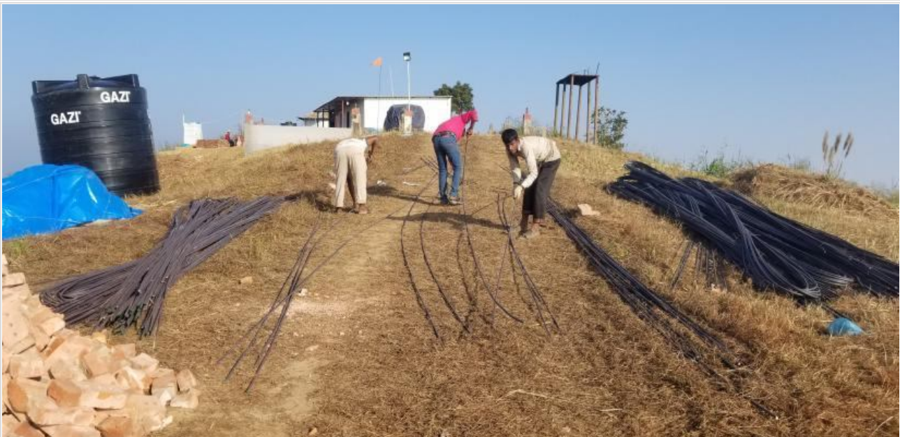
MS rod cutting & binding on 12-01-21
