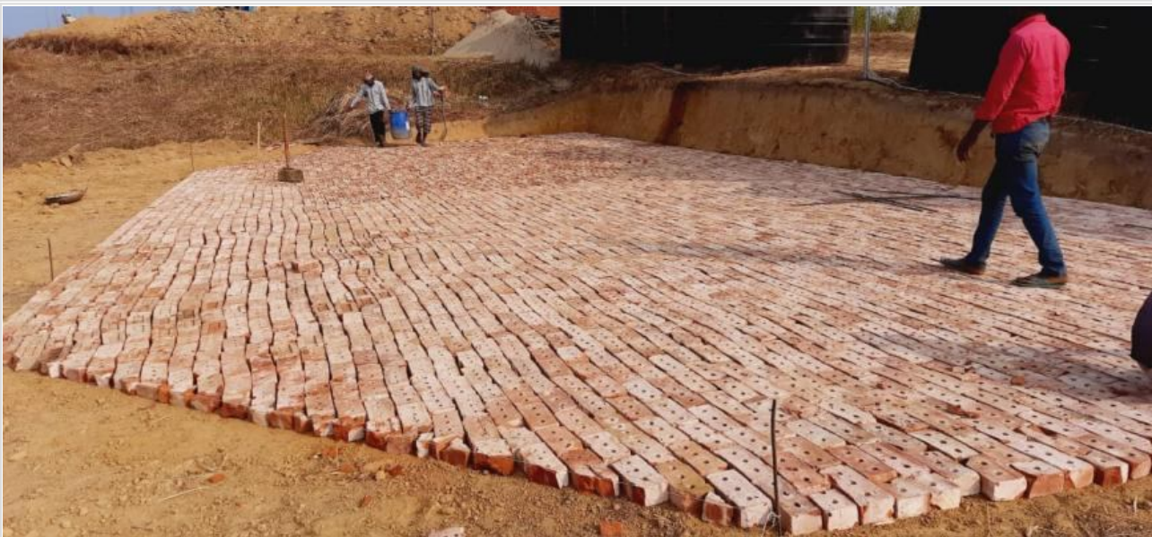
Soling for PVC Water Tank on 20-01-21
