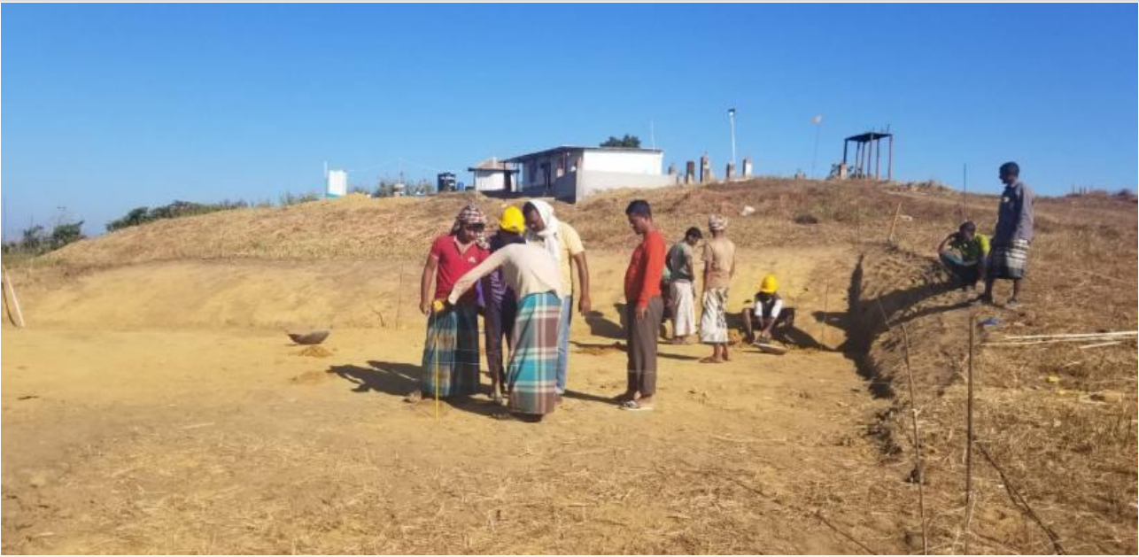
Guest House-Preparation for Layout on 07-01-21
